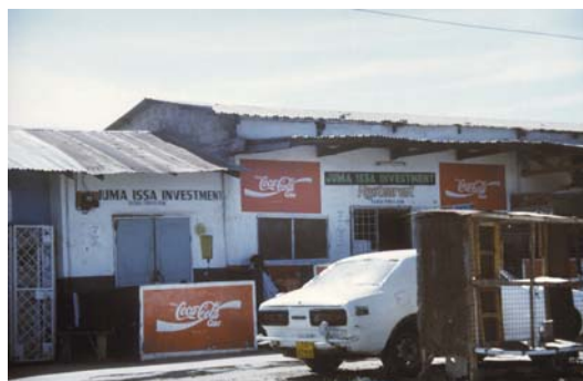
Fig 5.1 Manzese streetscape Dar es Salaam
